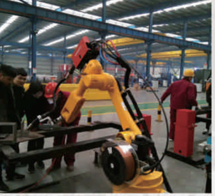
钢结构焊接应用 Welding application of steel structure
